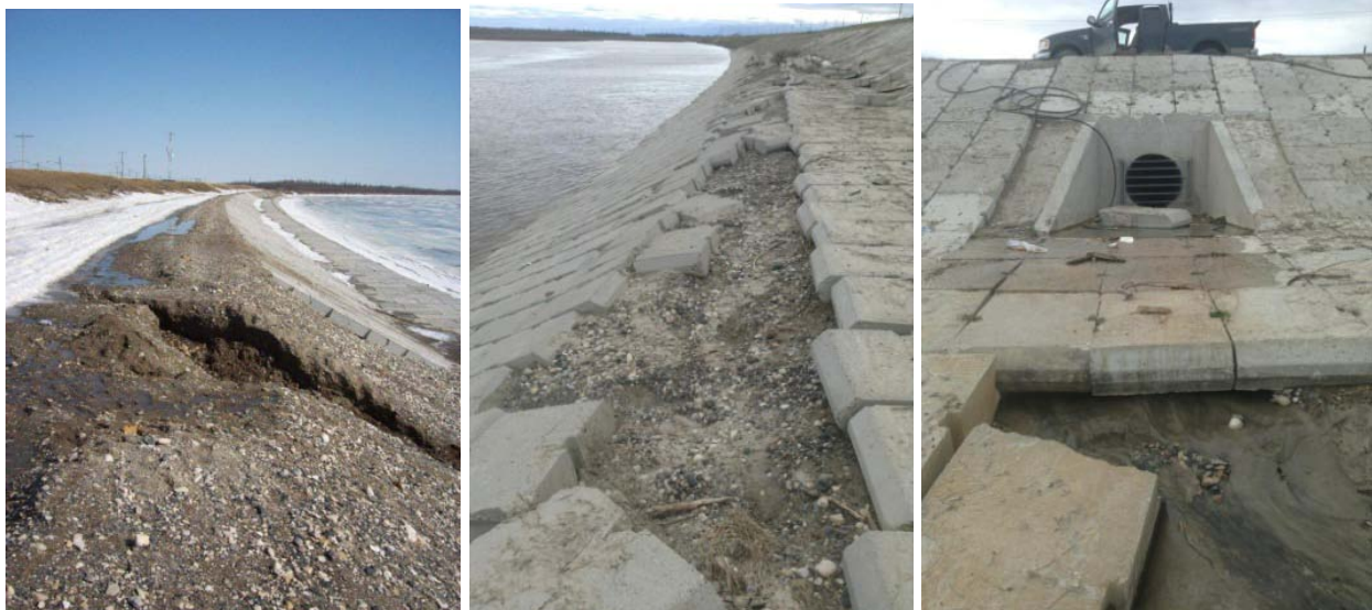
Figure 2-4: Examples of damage to the Stabilization Berm
