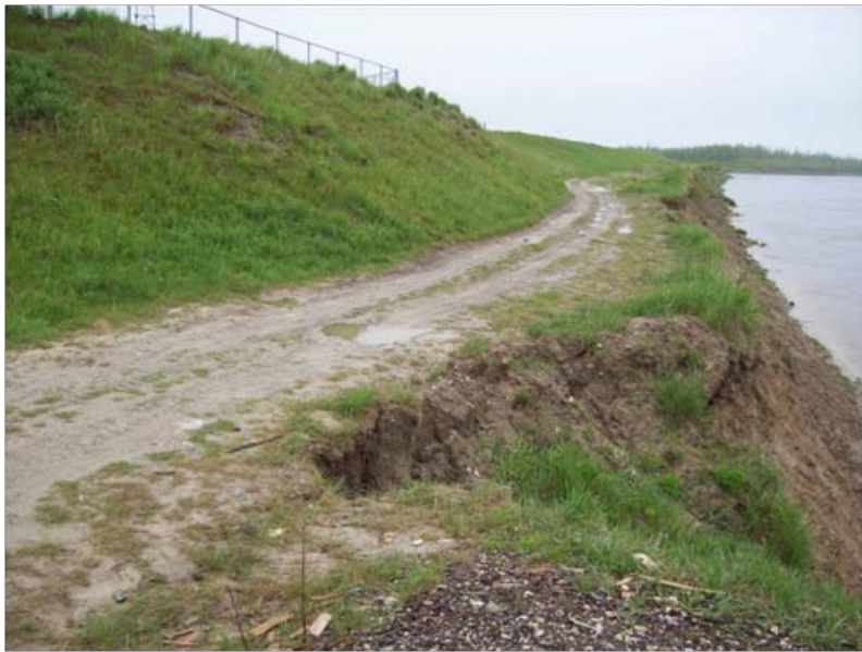
Figure 2-2: Example of ongoing erosion in 2008
